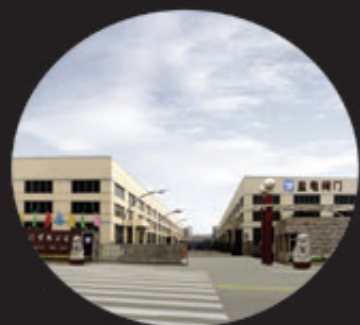
Gate Globe Check & Power Station Valve Plant
